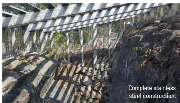
Completed Edison open cut cupola with bat-friendly 146-mm spacing between all steel members.
